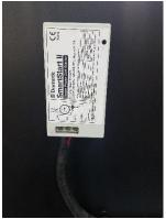
CORRECT (vertical surface, wires down, completely dry location)
