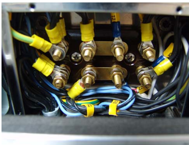
Fig. A.46: Generator power terminal box 120V/60Hz
