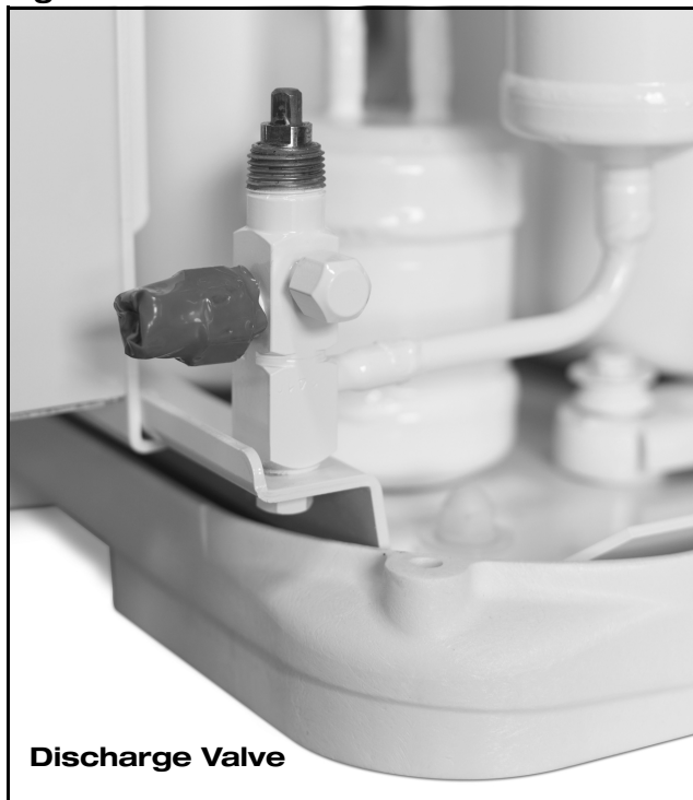
Figure 2: Service Valves Shown in Frontseated Position
