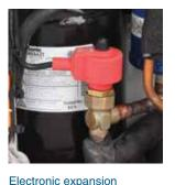
valve for precise control of superheat.
